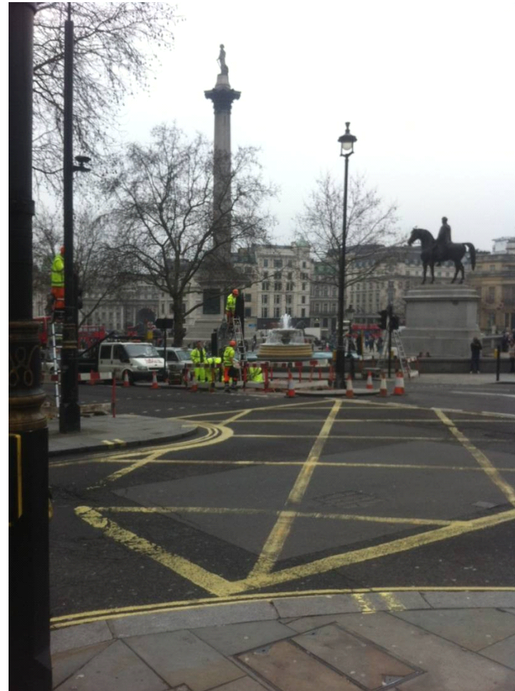
PC@TS installation works at Trafalgar Square
